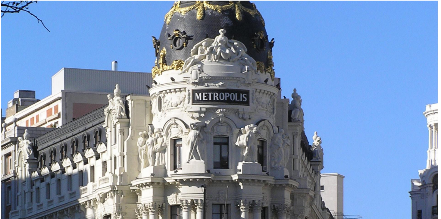
Metropolis building rehabilitation
