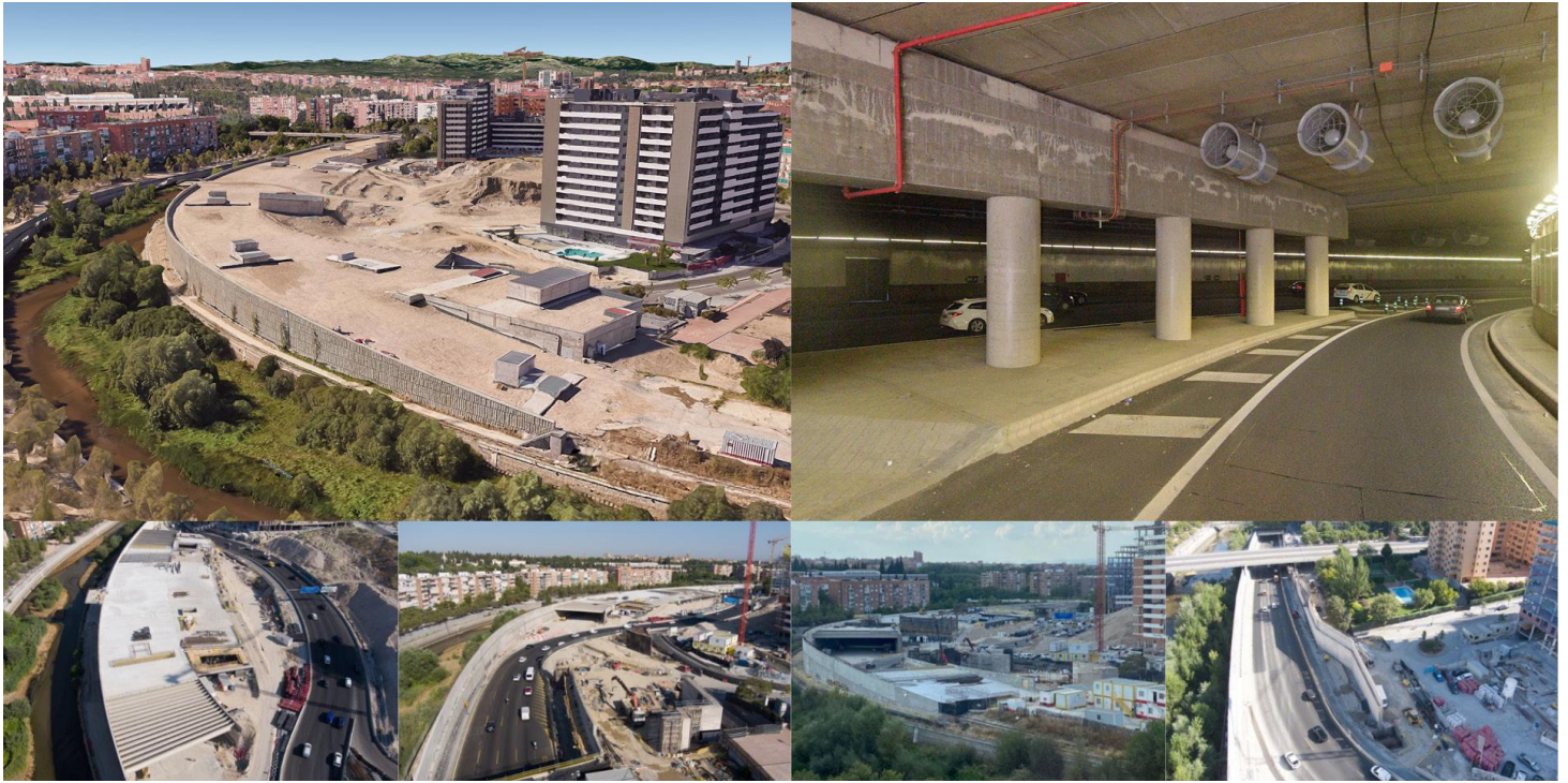
Pile foundation, Cast-in-place walls, Double T beams
