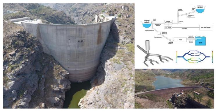
The Chira-Soria reversible pumped-storage hydroelectric power plant is an energy storage facility that features two water reservoirs at different elevations. Chira is the upper reservoir, while Soria is the lower one.
