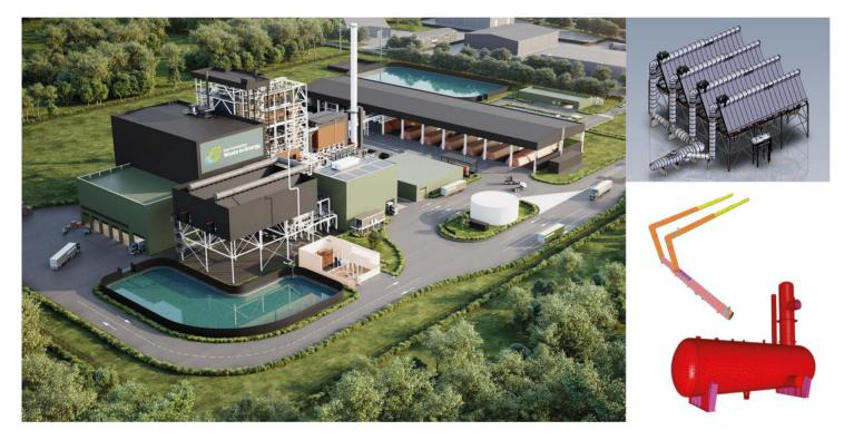
Air condenser ducts for the East Rockingham WtE plant 40 kilometres south of Perth in the state of Western Australia. The facility will recover thermal energy from 300,000 tonnes of municipal and industrial waste a year to generate 28.9 MWe of electricity, to be fed into the grid for supply to the agglomeration around Perth.
