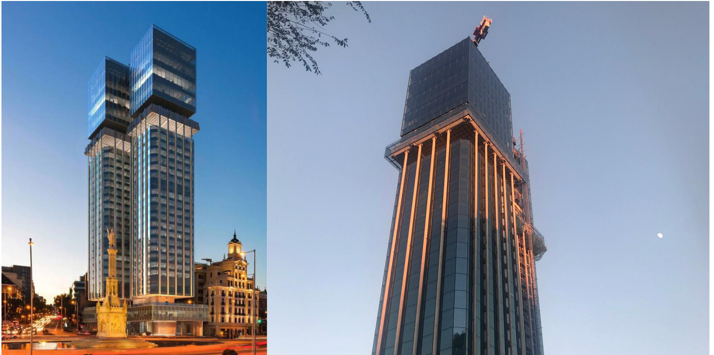
Cólon Towers rehabilitation
