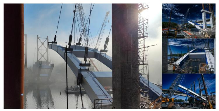
The new Pont Des Piles bridge is a 180 m span steel arch bridge with a relatively shallow rise. The deck consists of a composite section with double T steel beams and a concrete slab placed over them.
