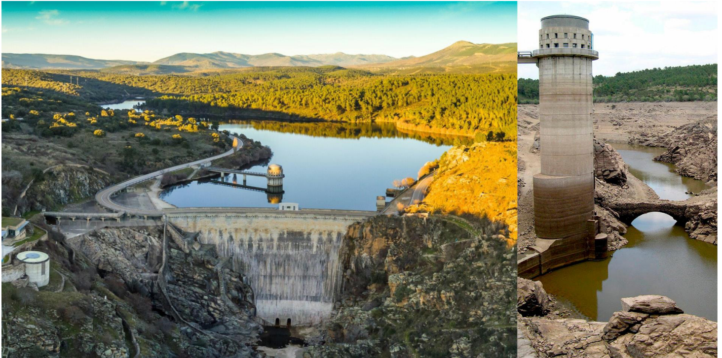
tower for controlling of reinforce concrete
