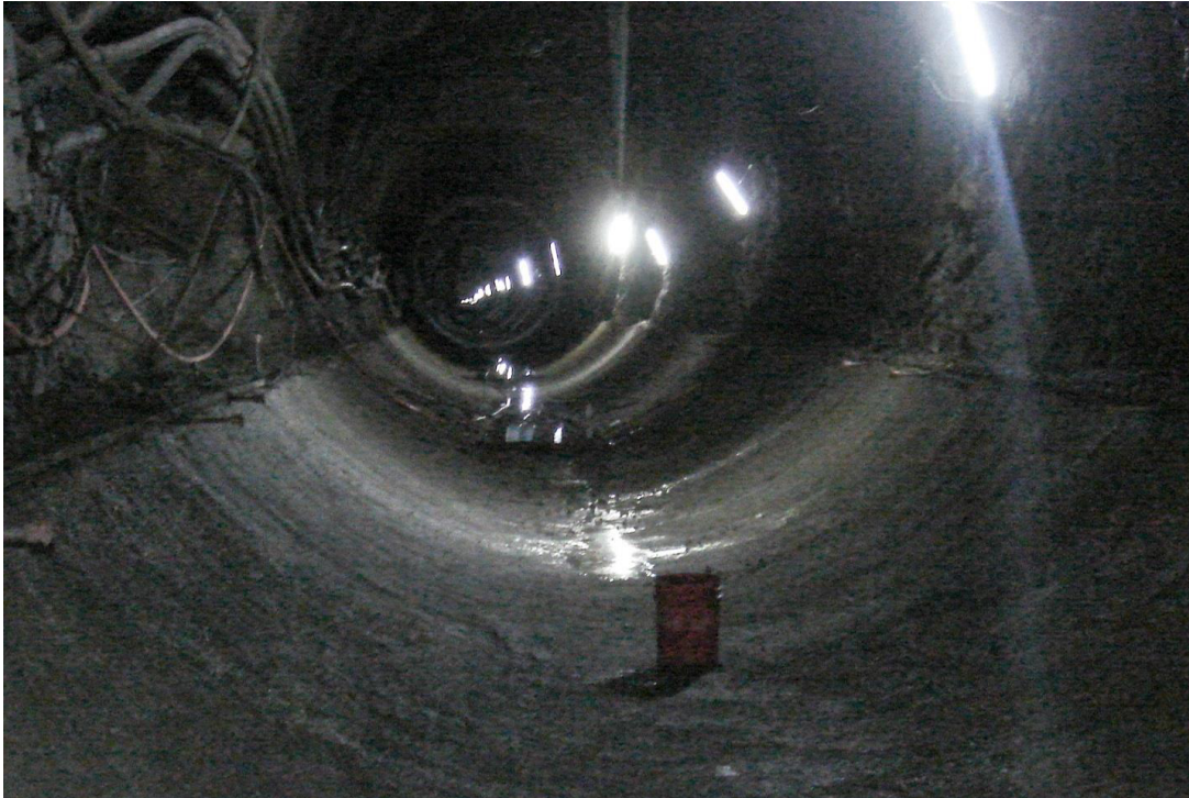
Reinforced concrete coat for the new headrace tunnel
