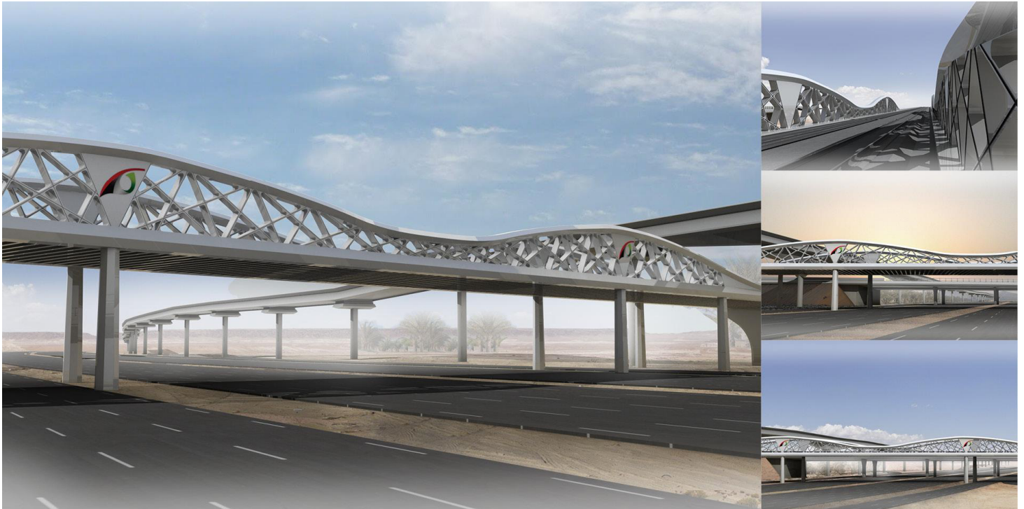
solution 1. Main bridge: truss of variable depth
