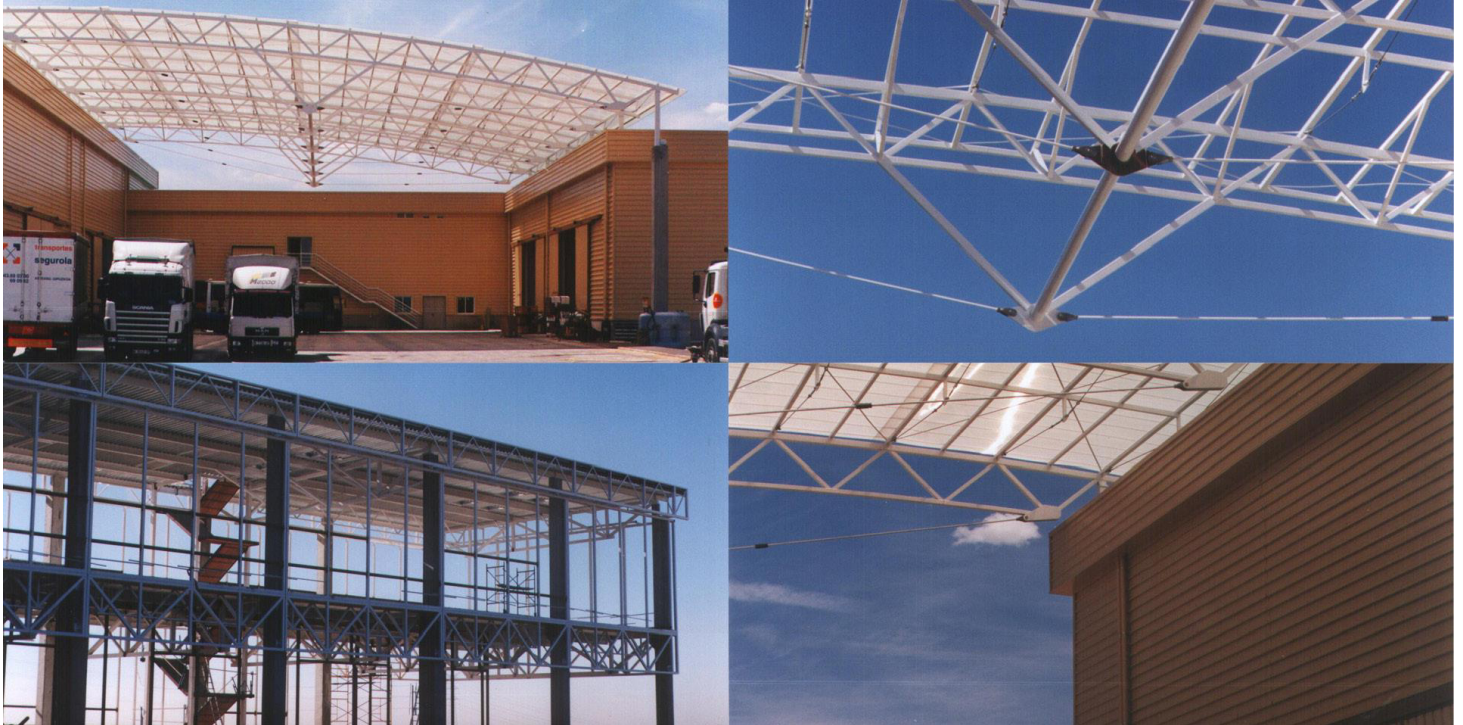
precast concrete columns and steel trusses roof
