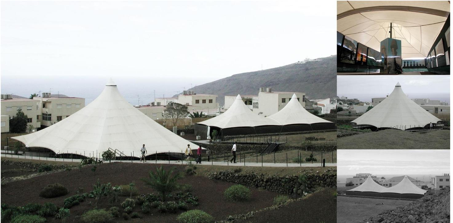
Membrana de PVC Ferrari Preconstraint 1002
