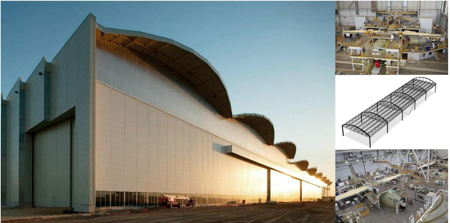
The assembly plant for the cargo plane A400M is composed by 9 modules, distributed in 2 hangars (4+5). They flank the block of the central building. Besides, there exists other auxiliary buildings who are part of the assembly plant. These are the painting workshop and other structure with lesser relevance, such as the pedestrian canopies, the access control building and one tower.
