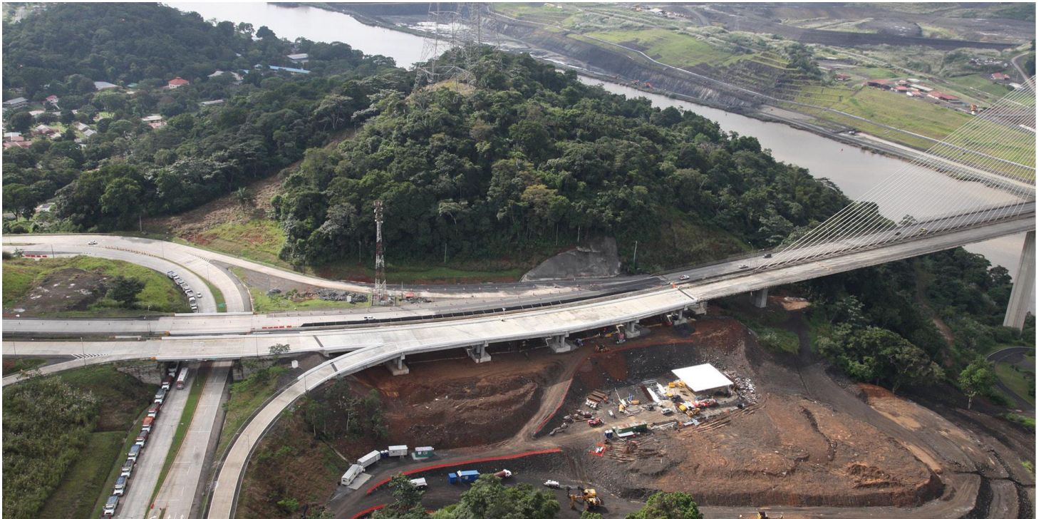
Northbound approach to the Centenario Bridge
