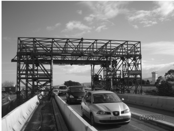
Figure 9. Travelling Formwork.
