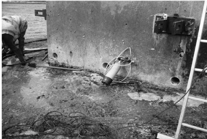
Figure 4. Strengthening of side pier foundations. Drilling operations
