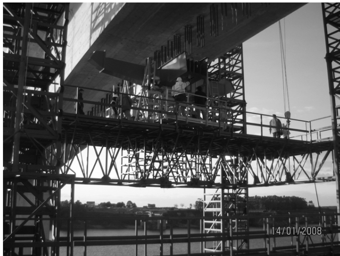
Figure 10. Placing of steel structure
