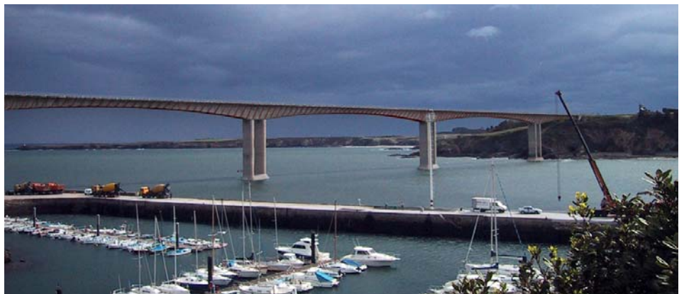
Figure 2.4 Los Santos Bridge [10]. Existing bridge comprising three 150,00 m spans, built by the cantilever method in the 1980's. The bridge deck was widened from 12,0 to 24,0 m by reinforcing the existing box cross section and using new ideas and materials in order to minimize the impact of the additional loads.
