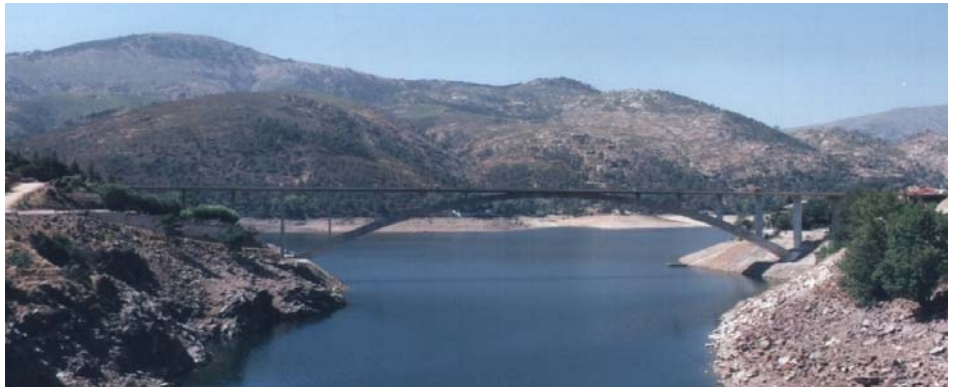
Figure 1.1 Before design and after construction [1]
