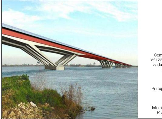
Structural Type: Composite main bridge with spans of 123.5m and 95.0m and approach viaducts 70.0m span, composed of prefabricated double-T girders Location: Carregado. Portugal Proprietor: Portuguese Ministry of Public Works Construction: Dragados-Sopol-Opca-Hagen Scope of Works: International tender for Construction Project and Technical Assistance
