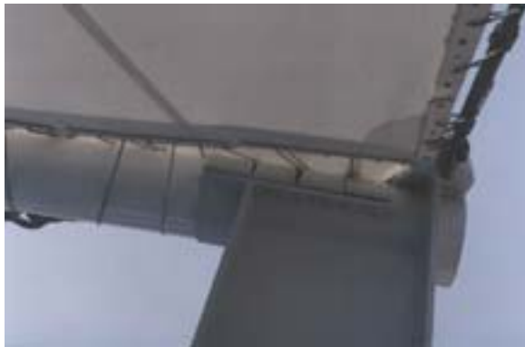
Photograph 8. Edge beam connection device.
