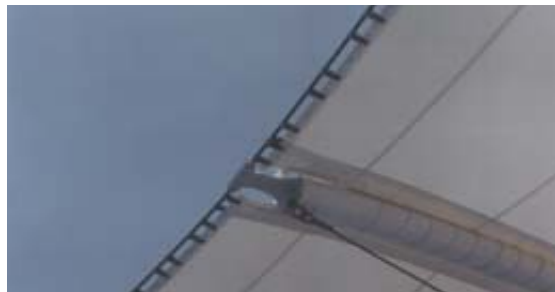
Photograph 7. Connection between cable and beam.
