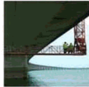
Structural Maintenance Engineering
